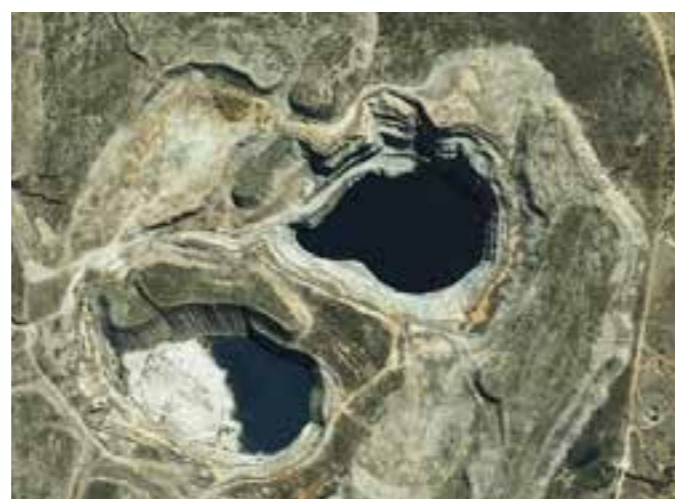
Photo: Old mining sites are ideal for PHES. For example Genex Power has issued a prospectus for a 330MW PHES system at a former gold mine in North Qld.
